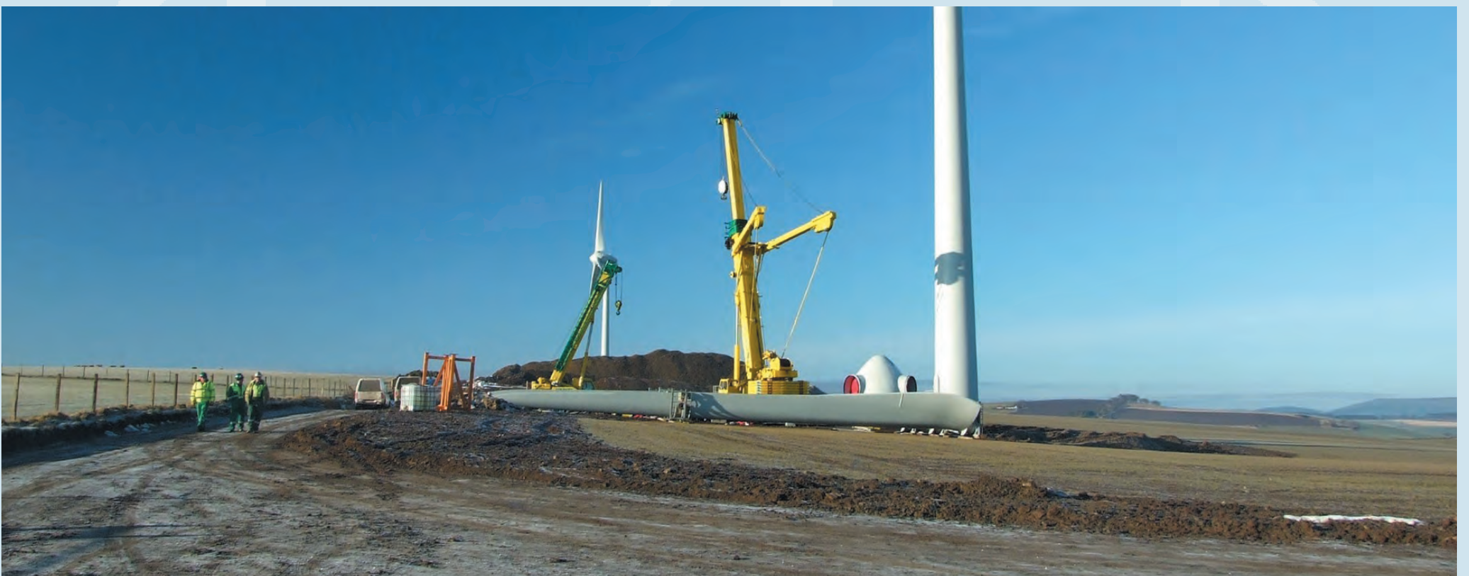
Construction of Newton of Fortrie Wind Farm in Aberdeenshire
